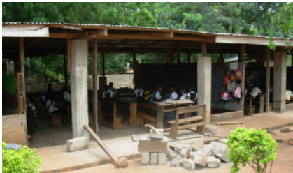
School structure being improved
