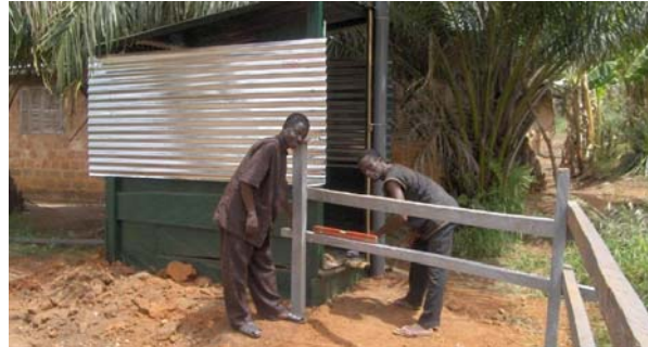
Constructing an outhouse and garden fencing
